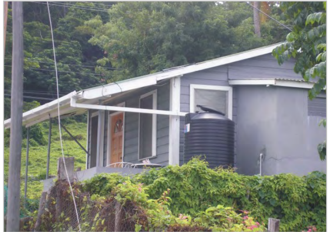
Household rooftop rainwater catchment systems in Carriacou.
