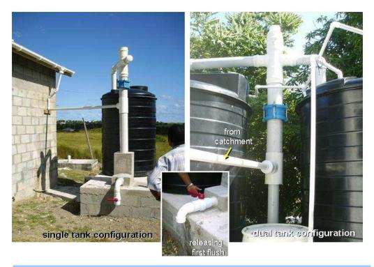
Figure 2 RWH demonstration models with new storage and first-flush diverters
