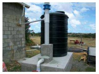
**Figure 13** Installed storage capacity and first-flush diverter
