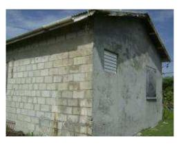
**Figure 11** Demo site before installation (note the rotten facia board and missing gutter section)
