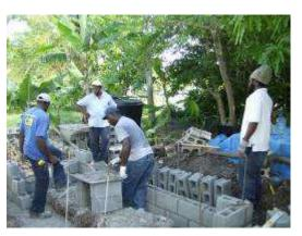
**Figure 9** Construction of the concrete tank platform
