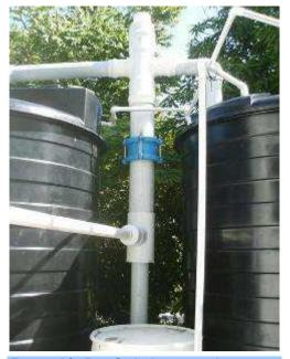
**Figure 10** First-flush diverter and new storage tanks
