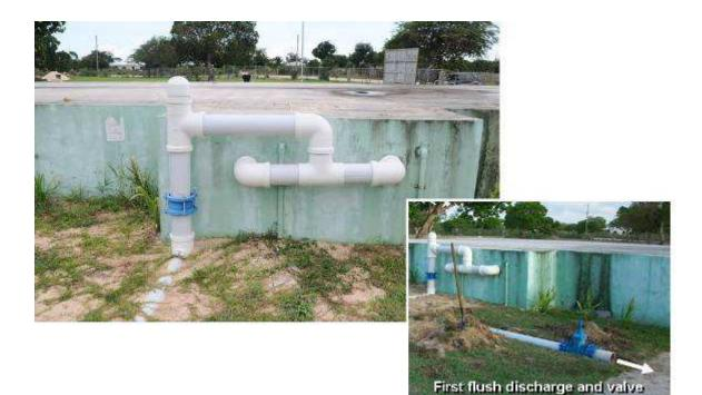
**Figure 17** Upflow first-flush diverter (left) and new inflow pipe configuration to cistern (INSET: discharge pipe from the first-flush)
