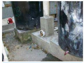
**Figure 5** Installation of the support base for the first-flush diverter
