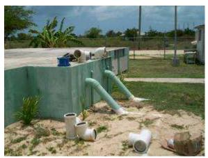
**Figure 16** Inlet pipes from roof catchments into cistern before installation
