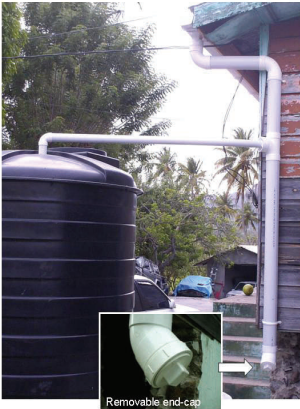
Figure 11 First-flush diverter
