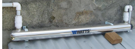
Figure 32 A typical ultra-violet lamp on a RWH installation (before entry to building)
