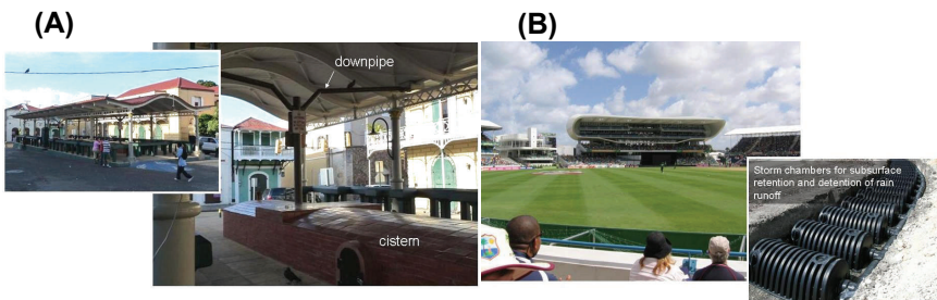
Figure 33(A) Rainwater capture from a municipal facility in Charlotte Amalie, St. Thomas, USVI; 33(B) Rainwater harvesting for irrigation of Kensington Cricket Oval, St. Michael, Barbados (runoff from field and roof catchments diverted to perimeter sub-surface drain - see inset) (Photos courtesy: Henry Smith and Andrew Hutchinson)
