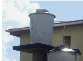
Figure 27: Typical header tank arrangement
