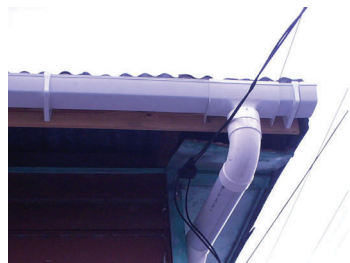
Figure 9 Typical PVC guttering and downpipe
