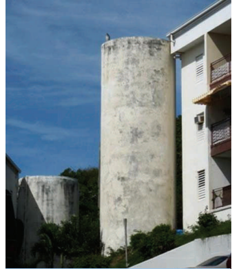
Figure 5 Cistern serving apartment building in St. Thomas, USVI. (Photo courtesy Henry Smith)
