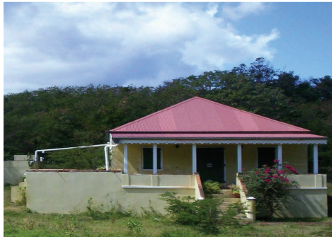
Figure 4 Domestic RWH system with cistern in St. Thomas (Source: H. Solomon and H. Smith, University of the Virgin Islands)
