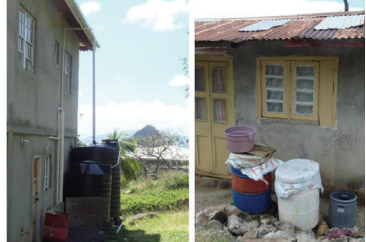
Figure 1 Typical household rainwater harvesting in the Caribbean
