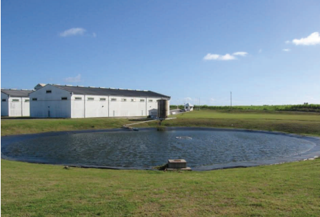
Figure 35 Rainwater harvesting diverted to surface storage at Mount Gay Distilleries, St. Lucy, Barbados; irrigation and firefighting purposes (Photo courtesy: Andrew Hutchinson)
