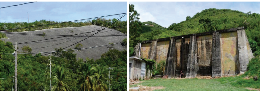
Figure 3 Old public water supply cistern and a hillside catchment surface both on St. Thomas, USVI (photos courtesy Henry Smith)
