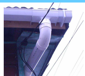
Guttering and downpipe
